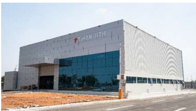
Figure 1: Mechanical Integration facility for UAV testing including control room
