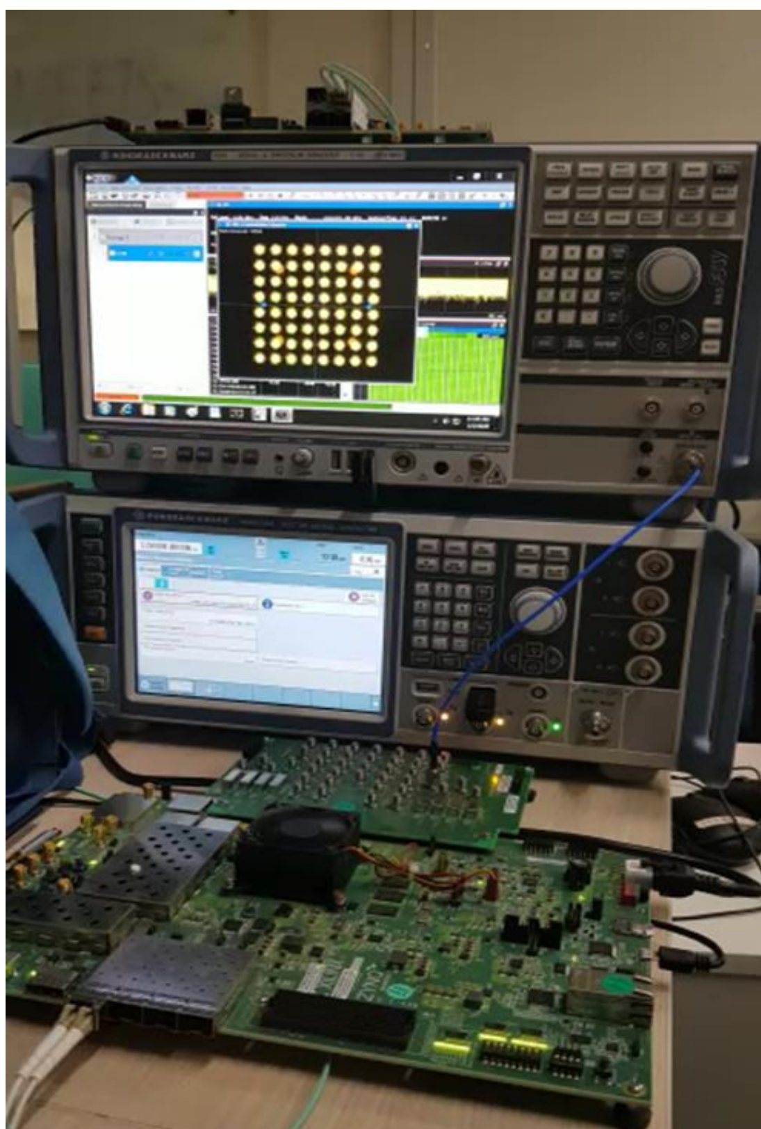
Fig. 4 5G Base Station Hardware
