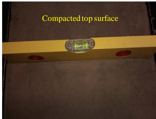
Fig 3.11 Level tube used to ensure level compacted surface
