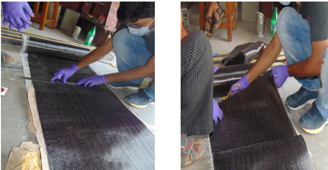
Figure 3.12 :Marking and Cutting of CF sheet
