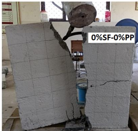
Figure 8. Failure of the panel without fibres
