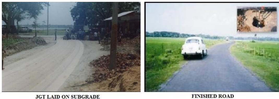
Figure 2.2 Section of road prior and after construction
