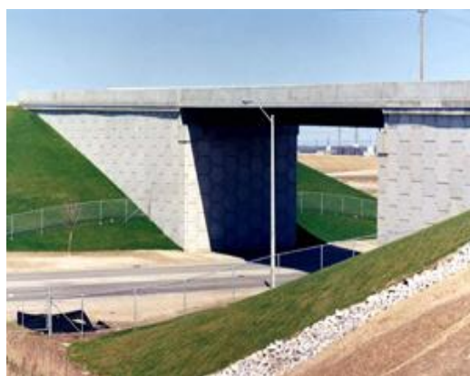
Figure 4.1: Bridge abutment of a Highway bridge
