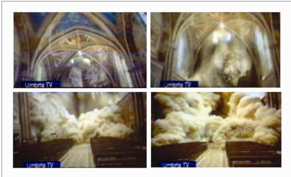
Figure 1.2: Photo sequence of the transept vault partial collapse occurred in the Basilica of Saint Francis in Assisi, Italy, during the Umbria-Marche earthquake (1997), Photo courtesy: [1].
