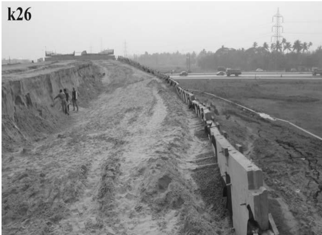
Figure 1.1: Failure during final stage of the embankment
