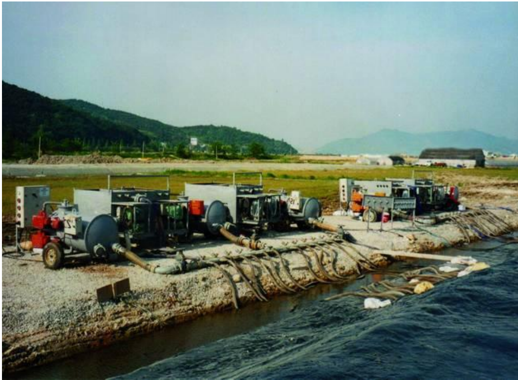
Figure 2.4: Vacuum consolidation to achieve the consolidation settlements
