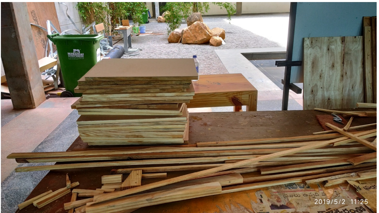
Fig1 63 Wooden pieces cut into frames
