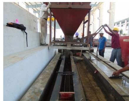
c) Placing of concrete
