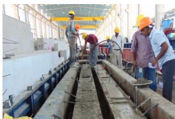
d) Compaction of concrete
