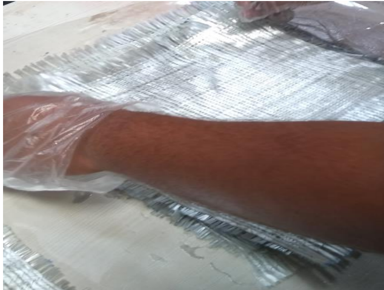
Figure 34 Placing of mat in plastic film
