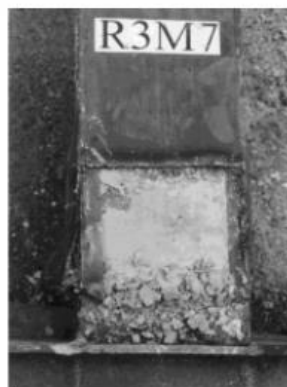
Fig.5 Typical concrete failure Appearances of Filled-in Concrete
