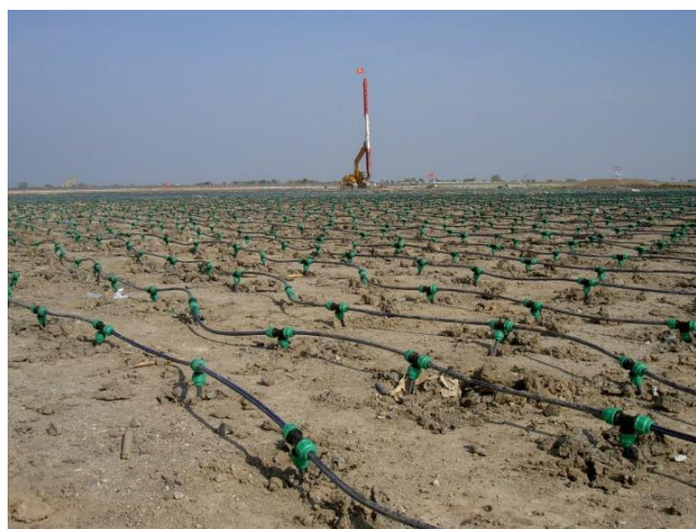
Figure 1.1: Vacuum preloading along with PVDs (Image courtesy: COFRA)
