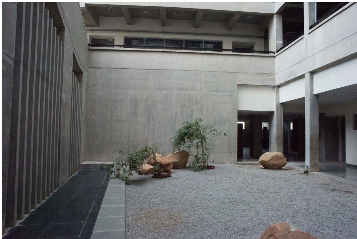
Figure 14: Courtyard wall, Ground floor, Academic Block
