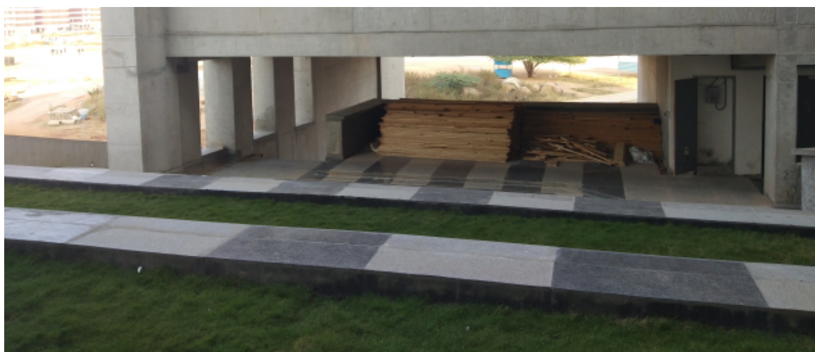
Figure 10: The initial site identified for installation
