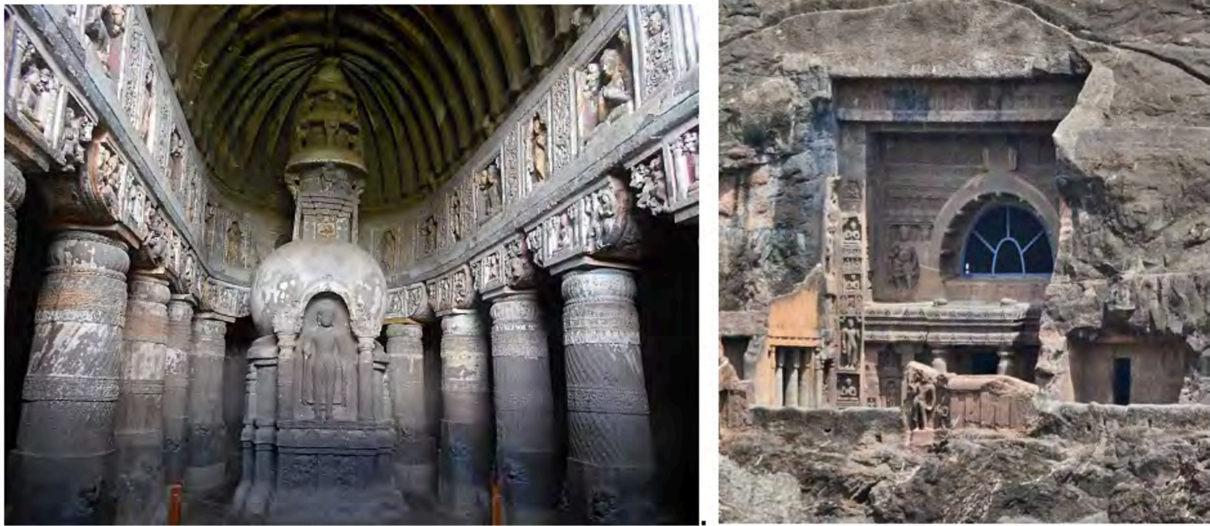
Entrance facade and inside worship hall cave 19
