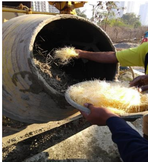
Figure 3. 3: Distributing fibers in concrete mix
