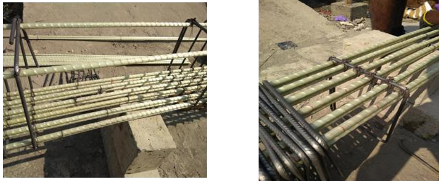
Figure 3. 4: Preparation of reinforcement cages with GFRP bars
