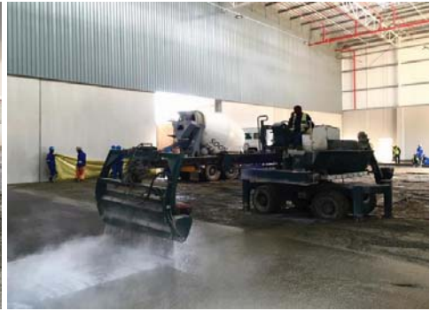
Figure.2: Topping Spreader, RSA @RCRIF
