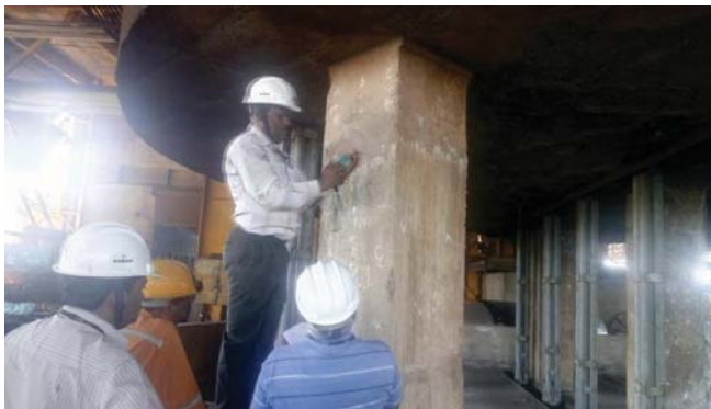
Figure 4: Rebound hammer test on a typical column
