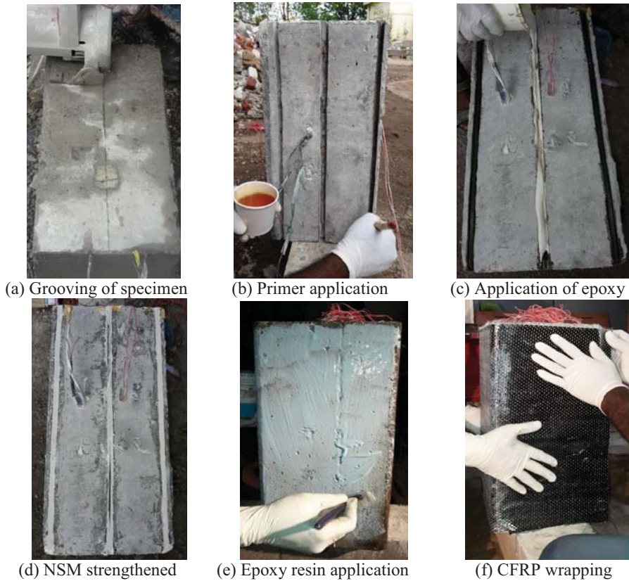
Figure 3: Systematic strengthening procedure for hybrid strengthening of RC column
