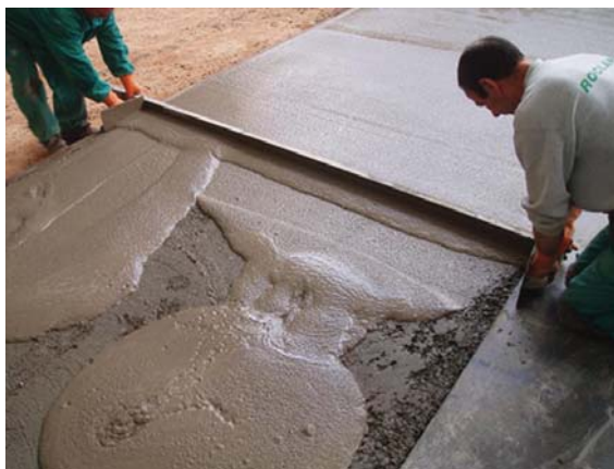
Figure. 10: Application of coloured wet on wet slurry, Spain @Suesco
