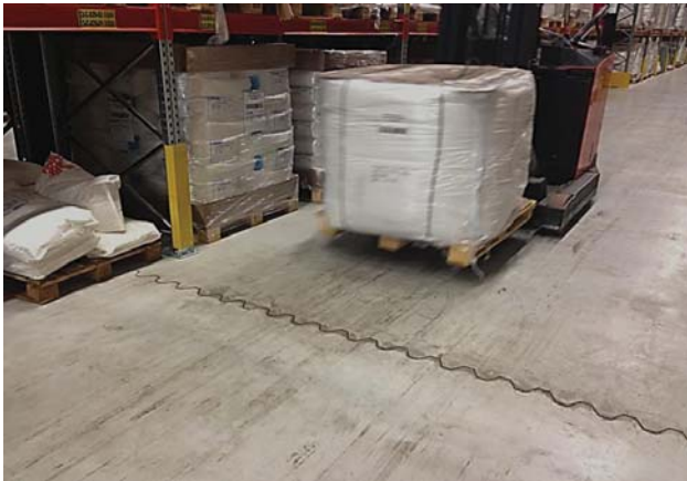
Figure. 5: Disruptive face joint – UK ®Permaban
