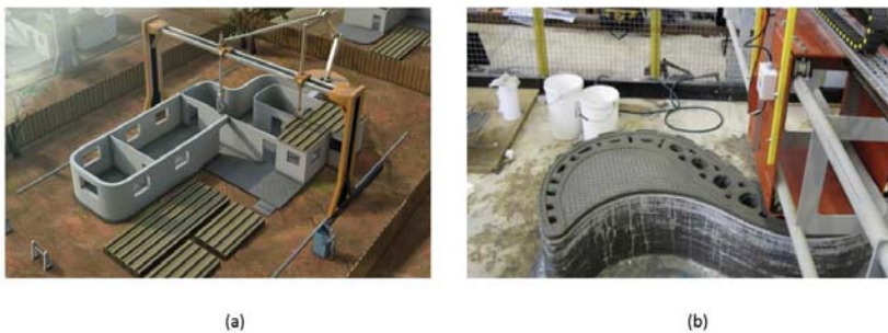
Figure 1. (a) Contour crafting (CC) [5] (b) Concrete printing processes [6]
