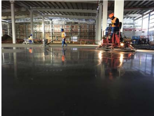
Figure. 7: VRS jointless floor, Peru @Pavimenta
