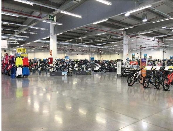
Figure. 9: 8-year-old light grey coloured surface hardener, Spain @Roeland
