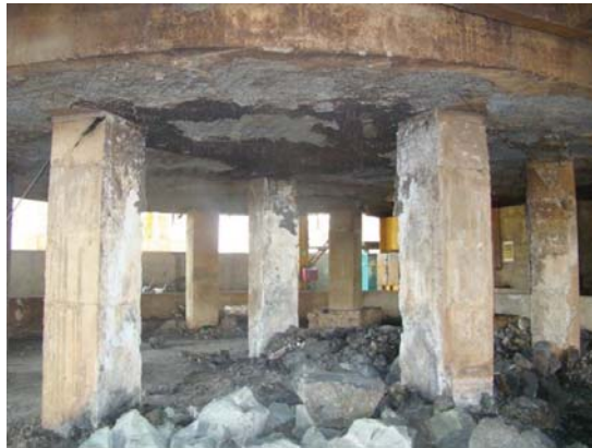
Figure 1: Photograph of furnace supporting structure
