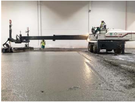
Figure.1: Laserscreed, Spain @RCRIF
