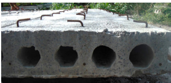
(a) Installation of Shear Keys
