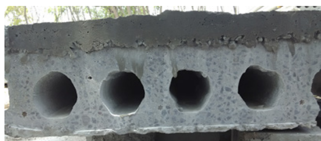
(b) Hollow Core Slabs with Bonded Overlay
