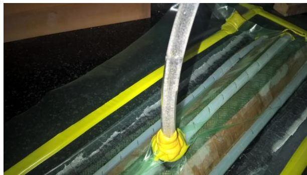
Figure 2.9: Resin filling the outlet tube
