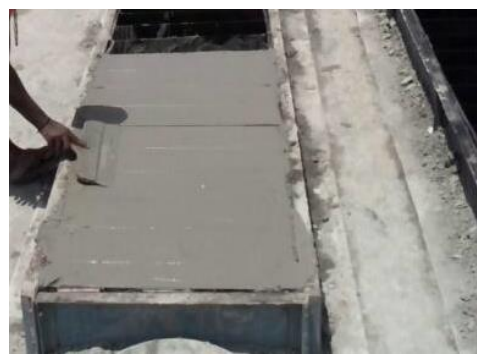
(c) Pouring in moulds
