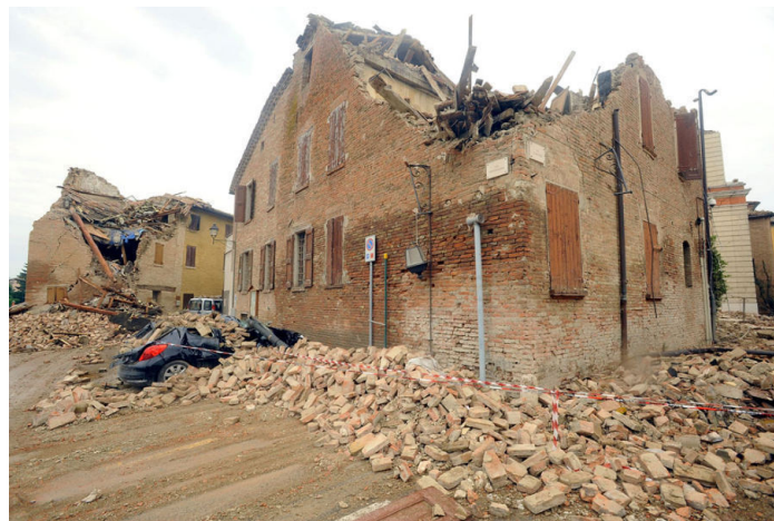
Figure 1.2: A earthquake-damaged building in Northern Italy ,in 2012 , Photo courtesyRoberto Serra/Iguana Press/Getty
