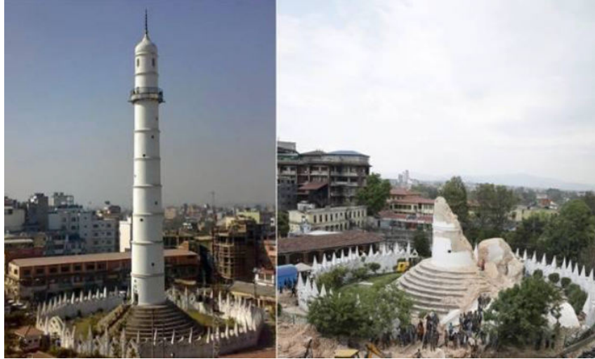
Figure 1.3: Daraharatower during Nepal earthquake Photo courtesy colinDaileda
