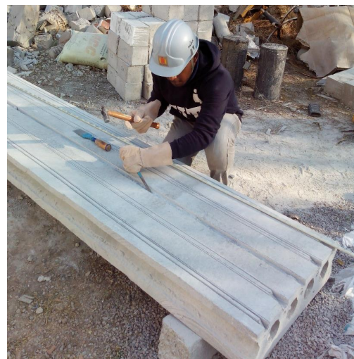
Chipping of grooves
