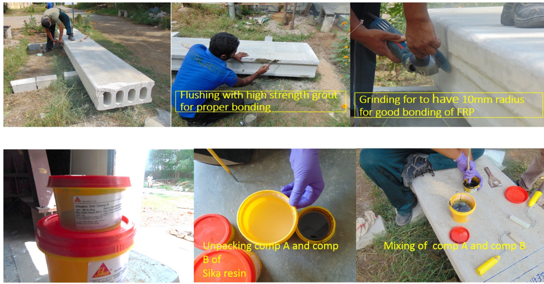
Figure 3.6: Surface Preparation and Epoxy Resin Preparation
