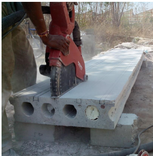
Cutting of grooves
