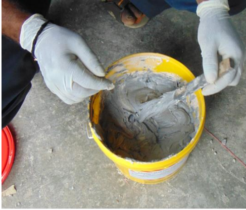
Mixing of Sikadur 30 epoxy
