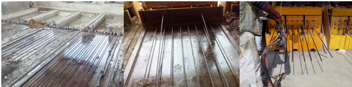
Figure 3.5: End block, Anchor and Hydraulic Prestressing Setup
