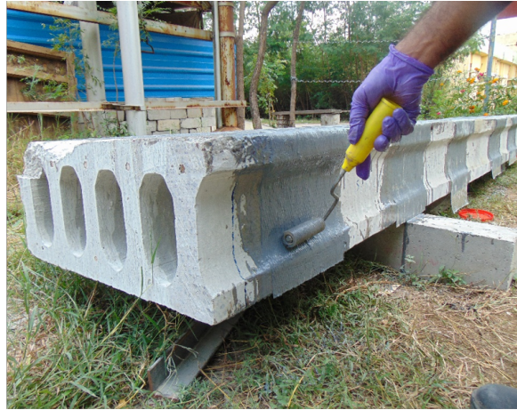
Use of Roller to remove entrapped air
