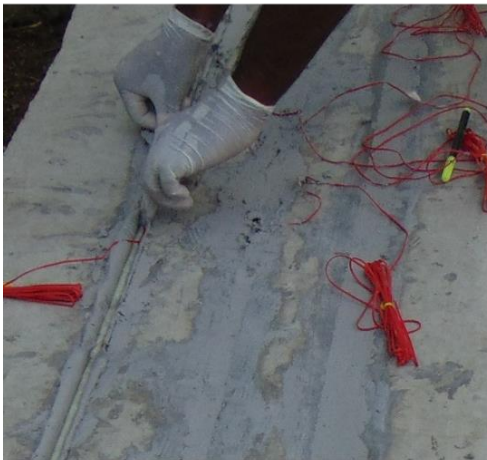
Application of GFRP bar
