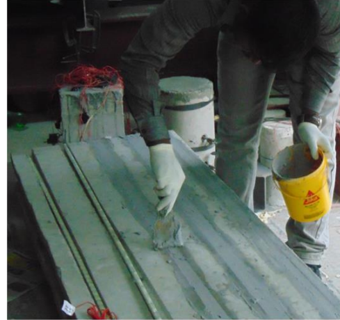
Surface levelled to concrete substrate
