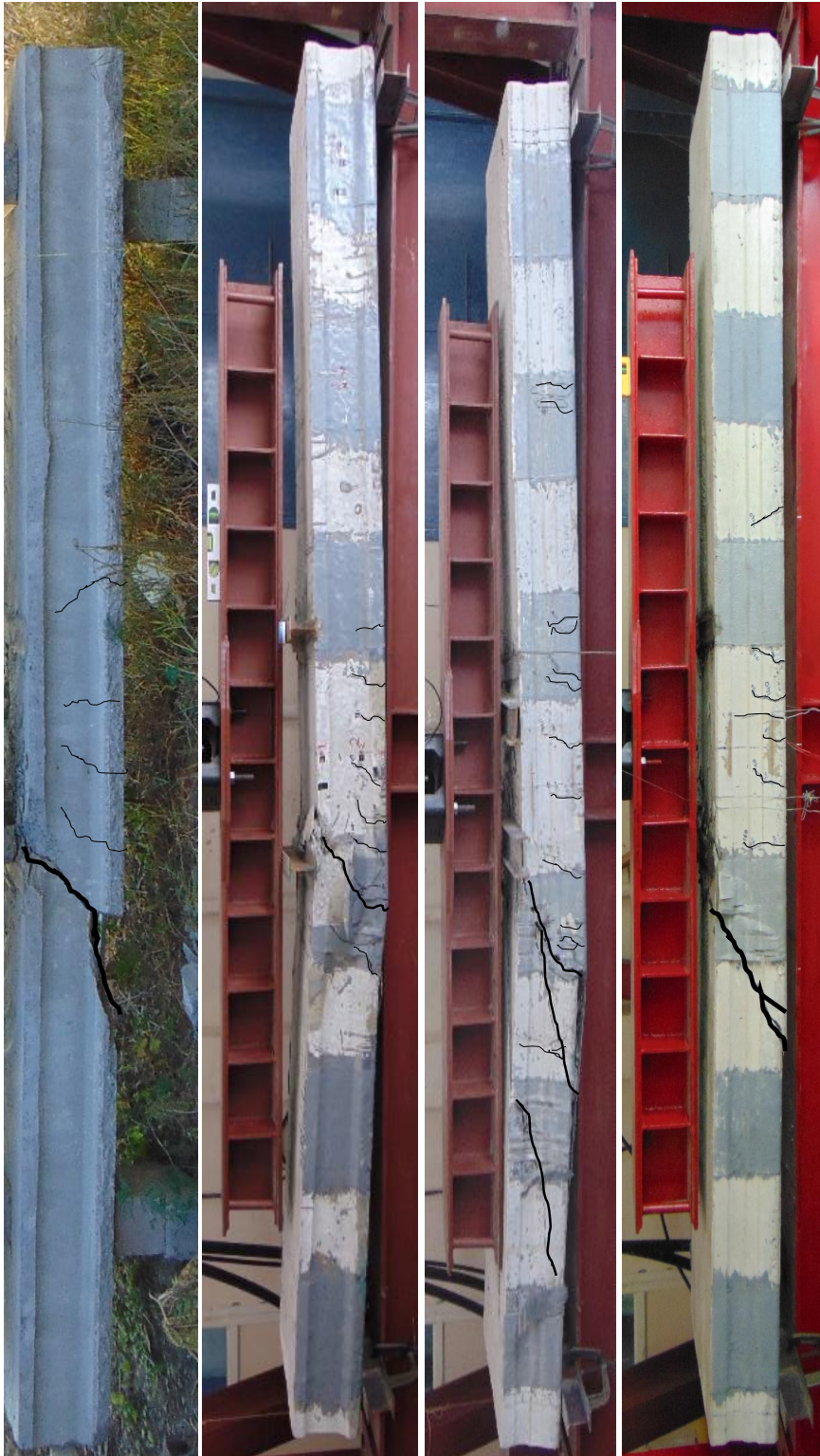
Figure 4.15: Crack Pattern at Failure - Series II
