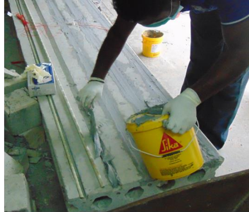
Half filling of grooves with epoxy
