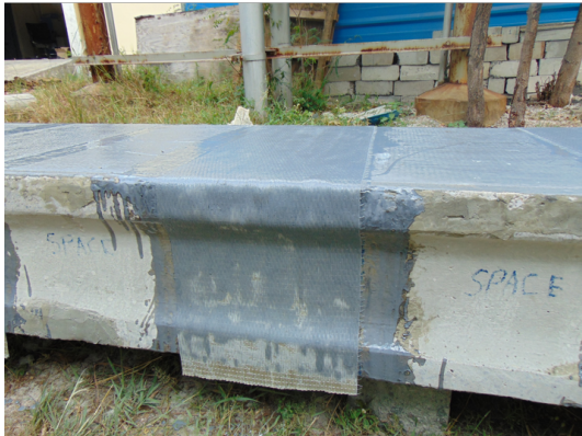
Shear Strengthening U wrap
