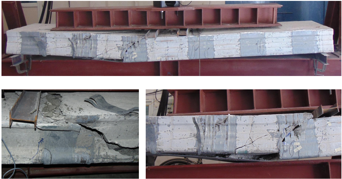
Figure 4.12: Mode of failure - II-S-250-5.4-EB-0.372-1.647
