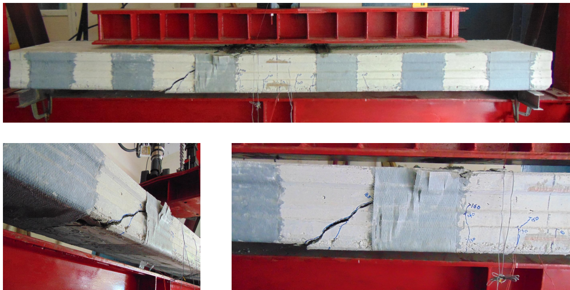
Figure 4.13: Mode of failure - II-S-250-5.4-EB-0.372-1.647
