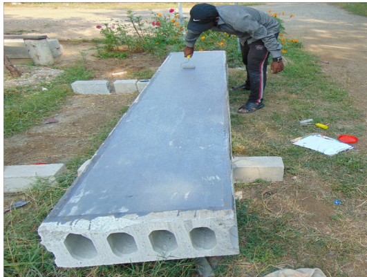
Use of Roller to remove entrapped air
