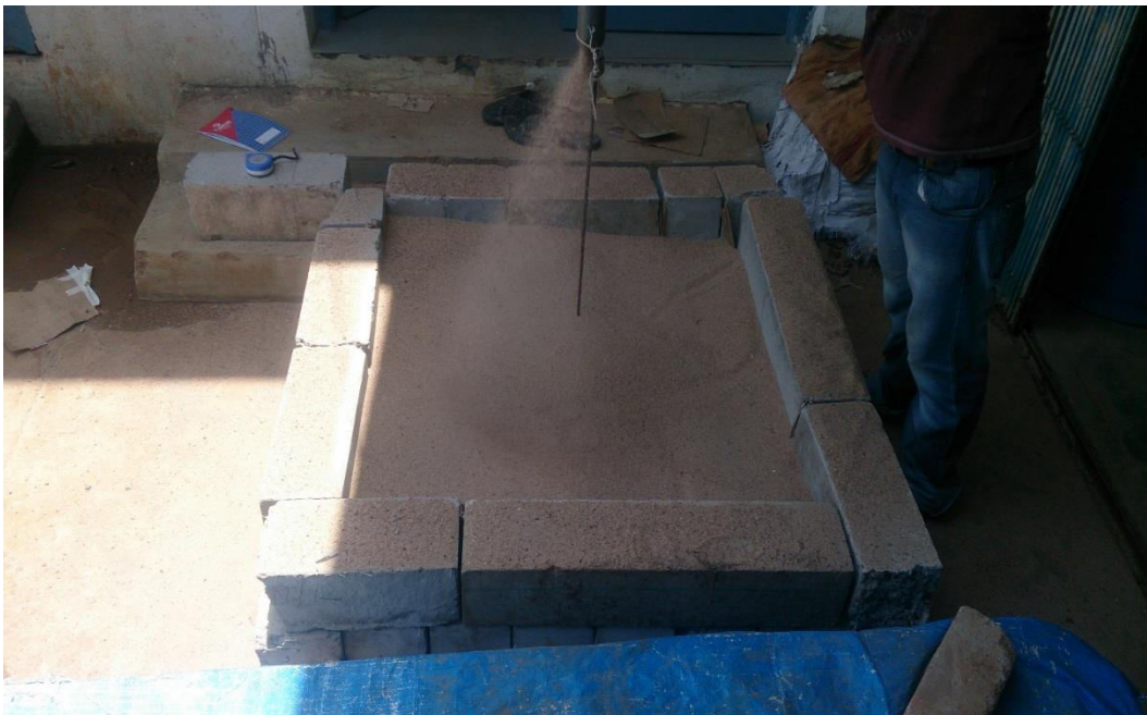
Fig.3.24: Filling of sand using pluviation technique
