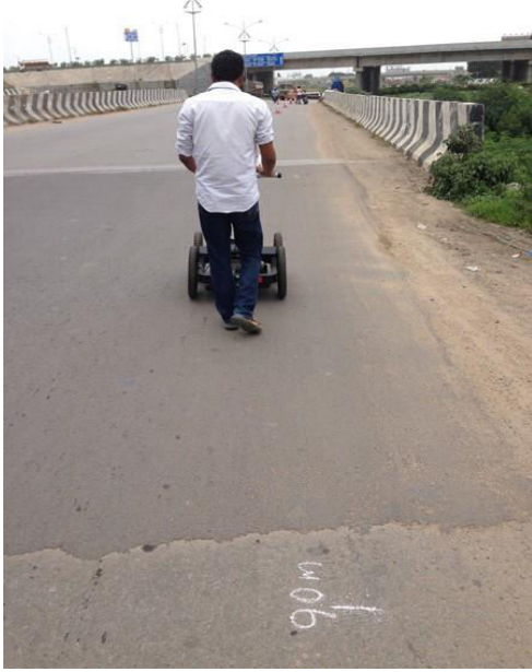
Fig.4.5: GPR testing on the pavement
