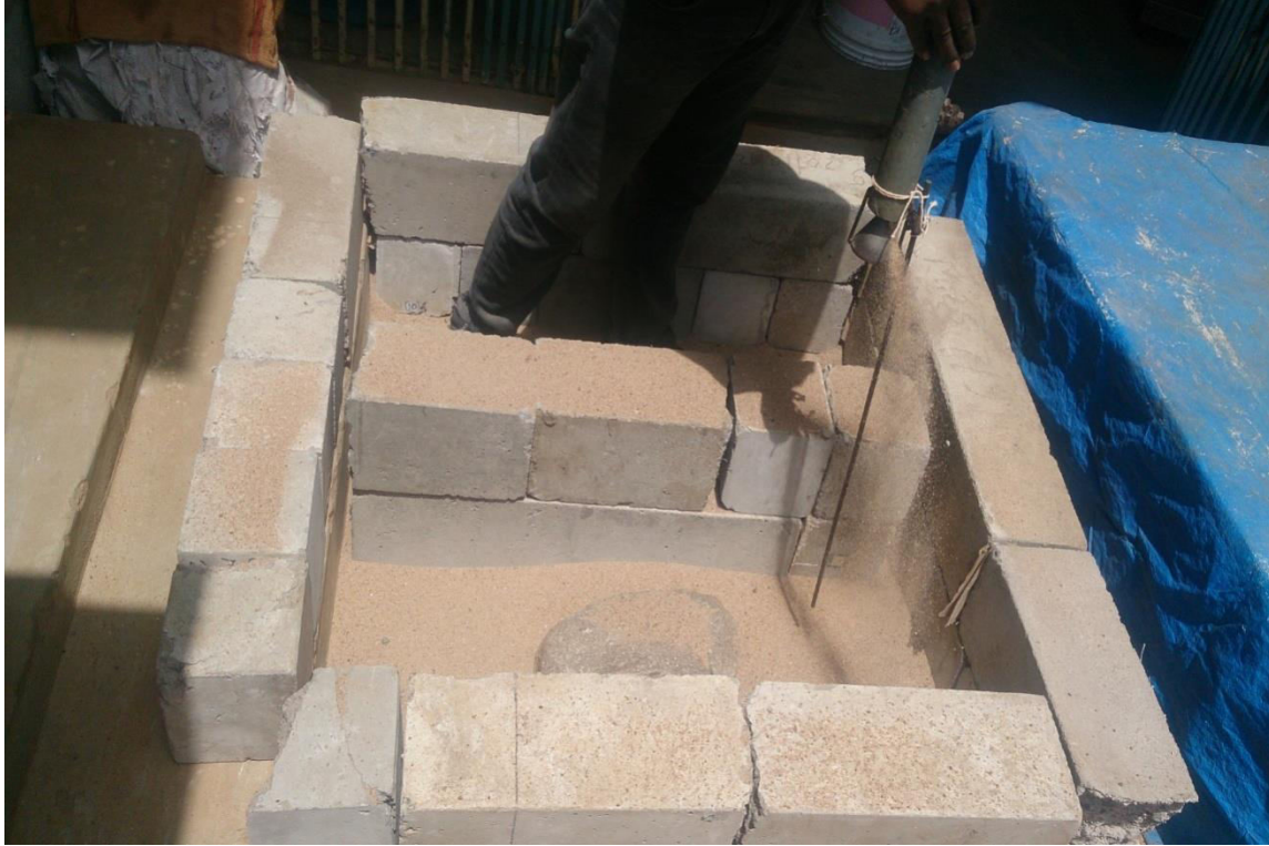
Fig.3.29: Test-pit showing sand being poured in the stone placed side
