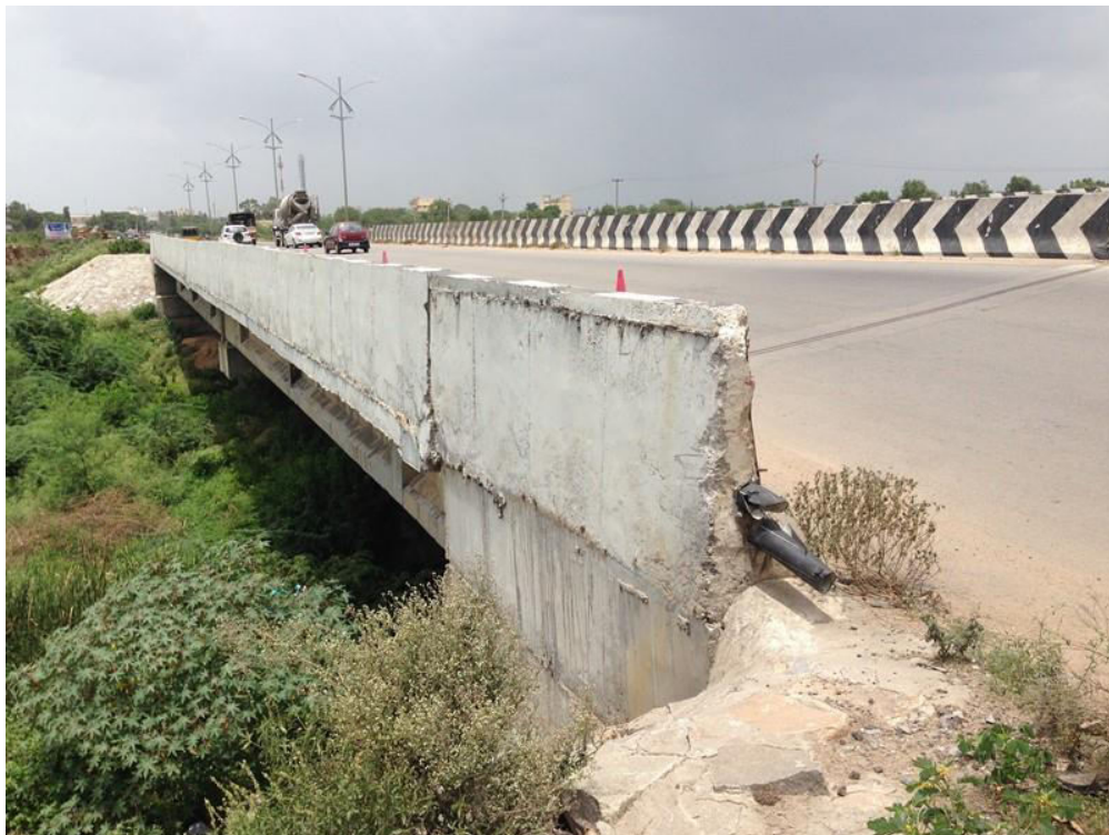
Fig.4.4: View showing the approach slab, wing wall and bridge deck
