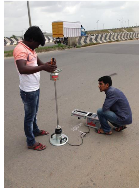
Fig.4.6: LWD testing on the pavement
