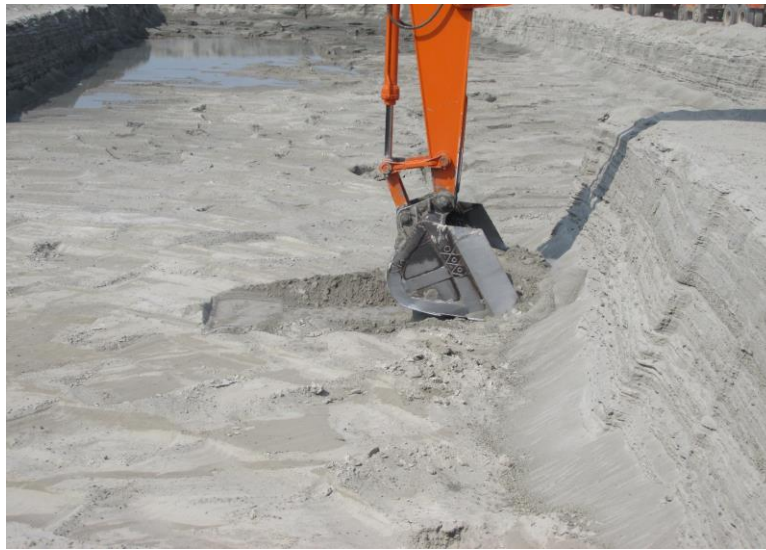
Figure 3.8: Collection of pond ash from RTPP using a back hoe
