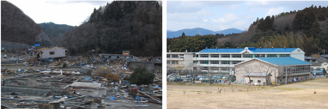
Figure 1.1: Affected sites after 2011 Tohoku Earthquake and Tsunami that impacted the existing ICT infrastructure. People took shelter at school building and had minimum access to rescue supply such as food, clothes, and medical treatment. ICT infrastructure was under constrained condition because of damages and slow recovery of land line cables.
