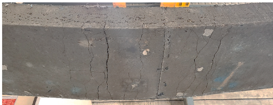
Fig. 10. Crack pattern on the tension side of FR-LWHCS (PO04).
